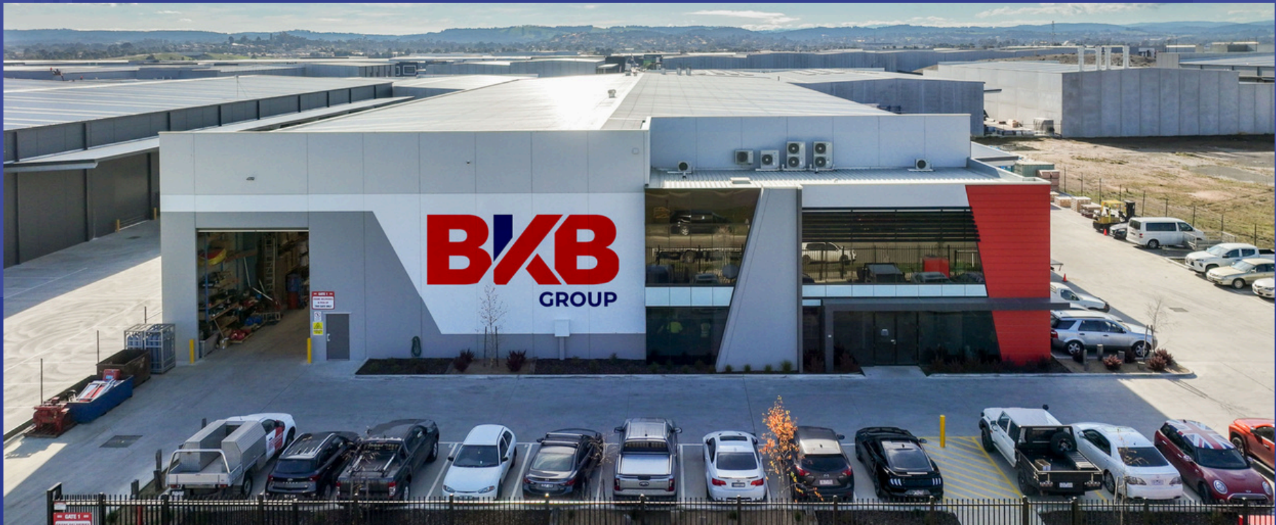
BKB MELBOURNE FACTORY & HEAD OFFICE
